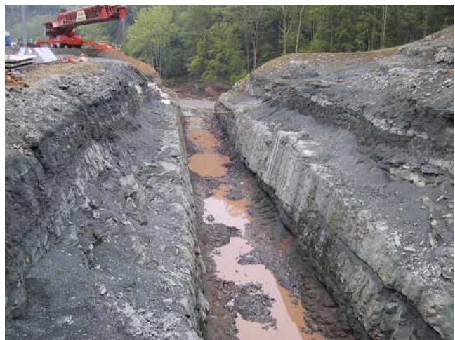
Figure 7-10 Presplitting in the bypass and auxiliary spillway at Hughes River Dam in West Virginia
