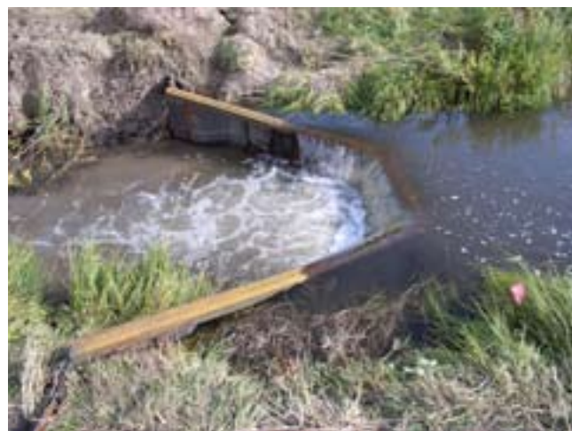
Figure 10 Sheet pile cross vane structure
