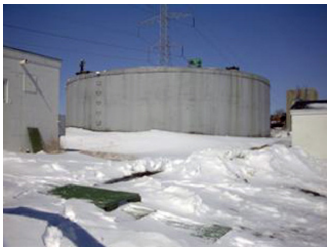
Figure 8 Continually stirred tank reactor (mixed digester)
