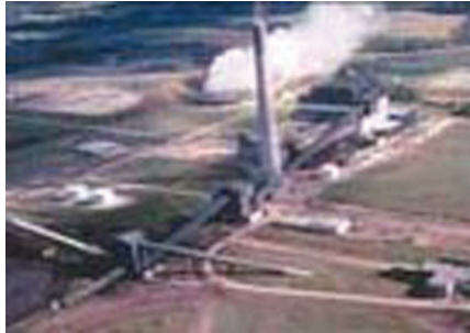
Coal-fired power plant
