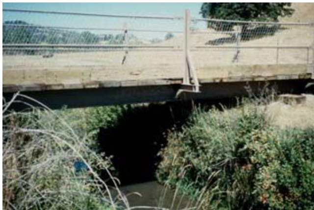
Figure TS14Q-1 Farm bridge with steel I-beam structural members and timber strip footing (Photo courtesy of Ben Doerge)
