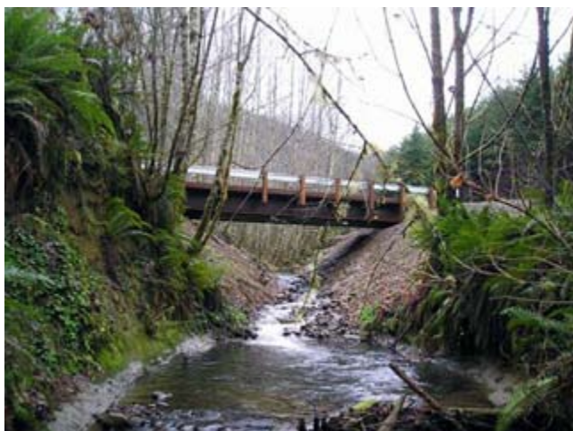
Figure TS14Q-4 Culvert replaced by bridge (Photo courtesy of Christi Fisher)
