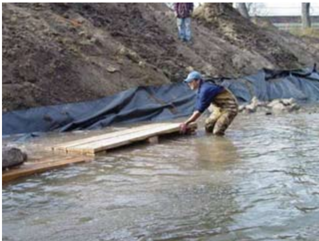
Figure TS140-1 (a) LUNKERS being installed as part of a bank stabilization project; (b) Completed LUNKERS project; LUNKERS are under the stone (Photo courtesy of Mike Martyn, USACE)
