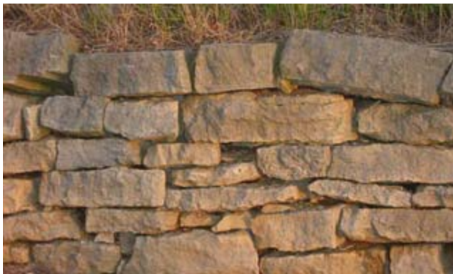
Figure TS14M-1 Dry stacked stone wall
