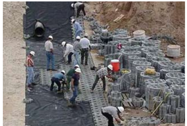
Figure TS14L-19 Hand placement of ACB blocks
