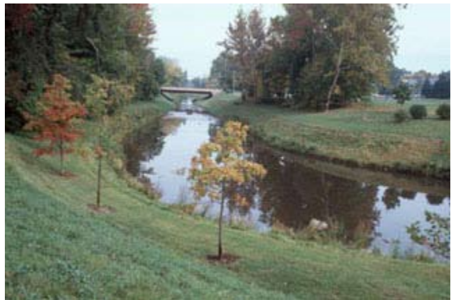
Figure TS14L-23 ACB revetment system 2 years after completion ( Photo courtesy of Joe Polulech )
