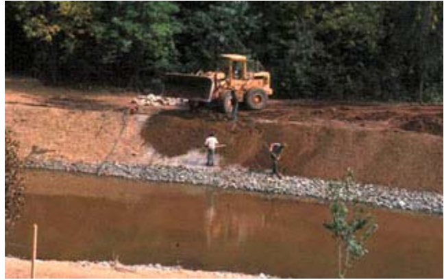
Figure TS14L-21 Filling ACBs with top soil ( Photo courtesy of Joe Polulech )
