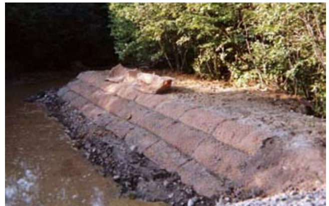
Figure TS14K–12 Vegetated gabions under construction
