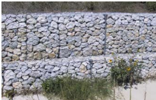
Figure TS14K–11 Gabions showing a neat, compact, placement of stone with a uniform appearance
