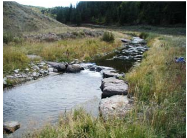
Figure TS14G-9 A J-hook grade control structure
