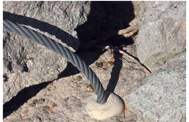
Figure TS14E-10 Wire rope anchored in boulder with epoxy
