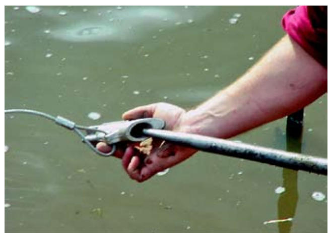
Figure TS14E-2 Drive rod being inserted into Duckbill ® anchor prior to installation
