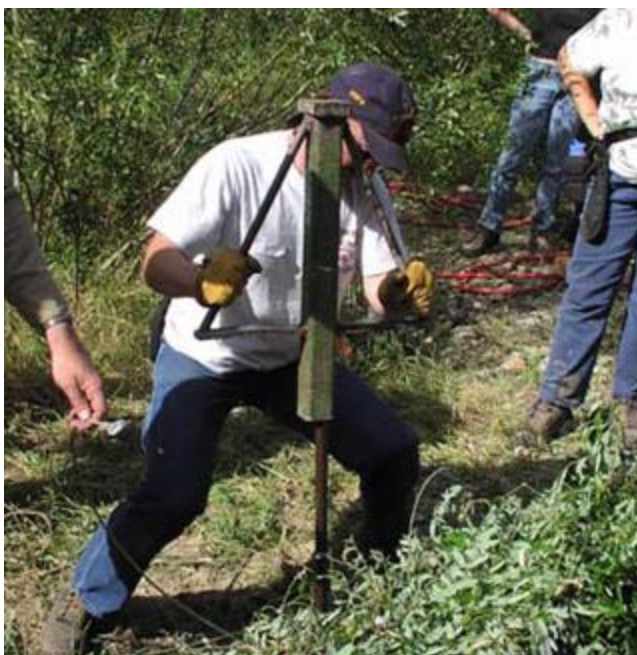
Figure TS14E-3 Post driver being used to install soil anchors
