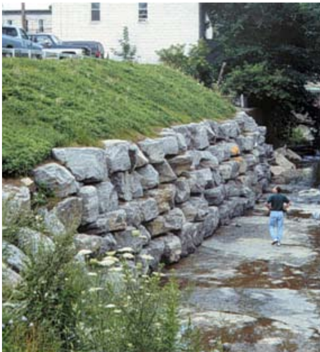
Figure TS14D-15 Reinforced soil slope with rock face (Photograph courtesy of Frank Cousin, NRCS MI)
