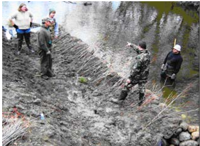
Figure TS14C-4 Toe of the slope lined with stone to control erosion
