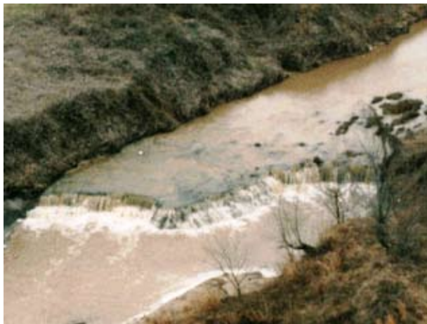
Figure TS14B-7 Headcut migrating upstream through cohesive streambed toward bridge in north-central MS. Headcut was triggered by downstream channelization.
