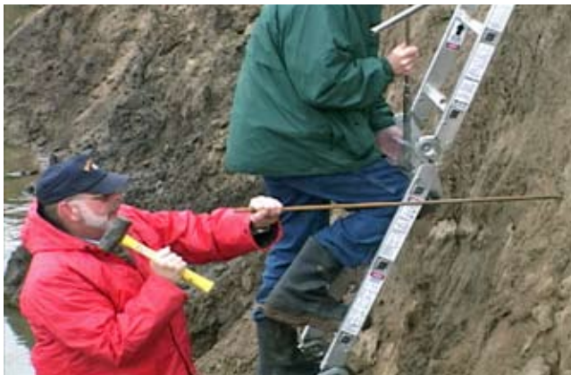
Figure CS9-17 Installing bank erosion pins
