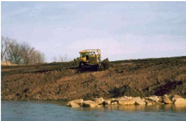
Figure CS9-8 Bank shaping with bulldozer
