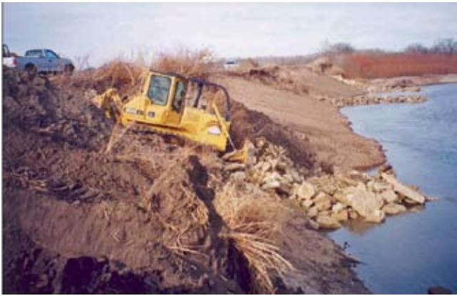
Figure CS9-6 Building weir on site 28
