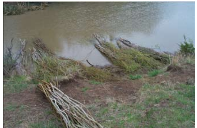
Figure CS9-13 Willow cuttings soaking in ponds
