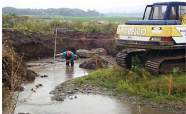
Figure CS7-4 Installation of a J-hook vane, Spafford Creek, NY
