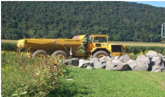
Figure CS7-3 Equipment and rock used for construction, Spafford Creek, NY
