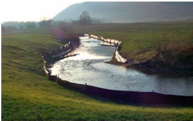
Figure CS7-6 Completed section of streambank stabilization, Spafford Creek, NY
