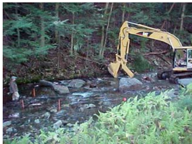
Figure CS6-9 Staking out a cross vane
