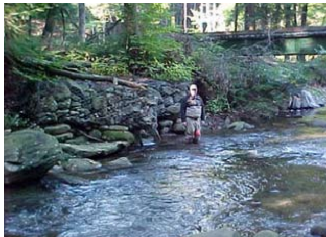
Figure CS6-4 Most downstream PennDOT bridge on Big Bear Creek
