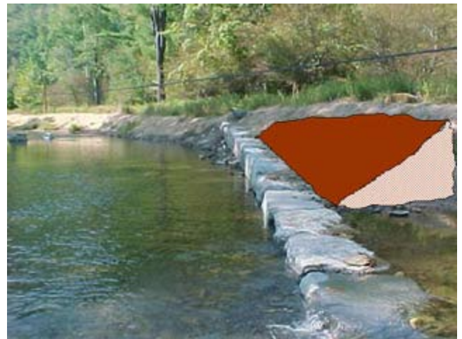
Figure CS6–18 Schematic representation of the improper fill technique on the upstream side of the vane
