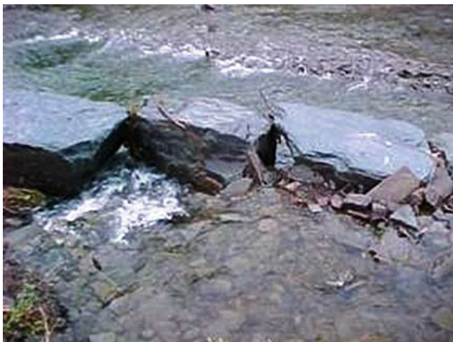
Figure CS6–14 Gap holes, which in high flow, become suck holes
