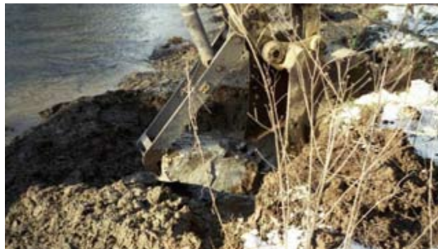
Figure CS6-13 Setting a footer rock (upstream direction is to the right)
