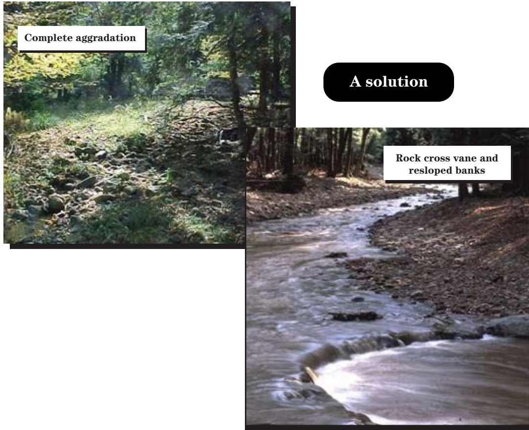
Figure CS6-21 Treatment of a channel avulsion with rock structures
