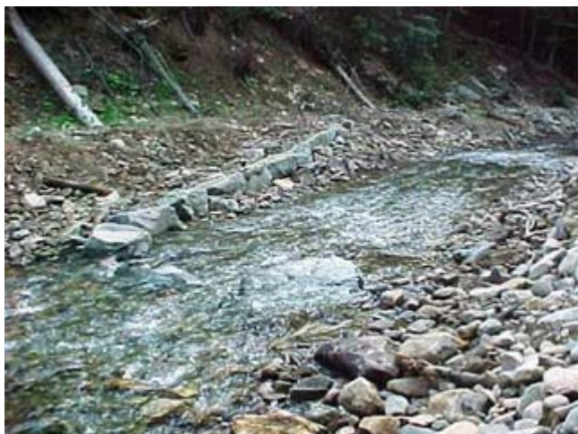
Figure CS6-7 J-hook rock vane on Big Bear Creek
