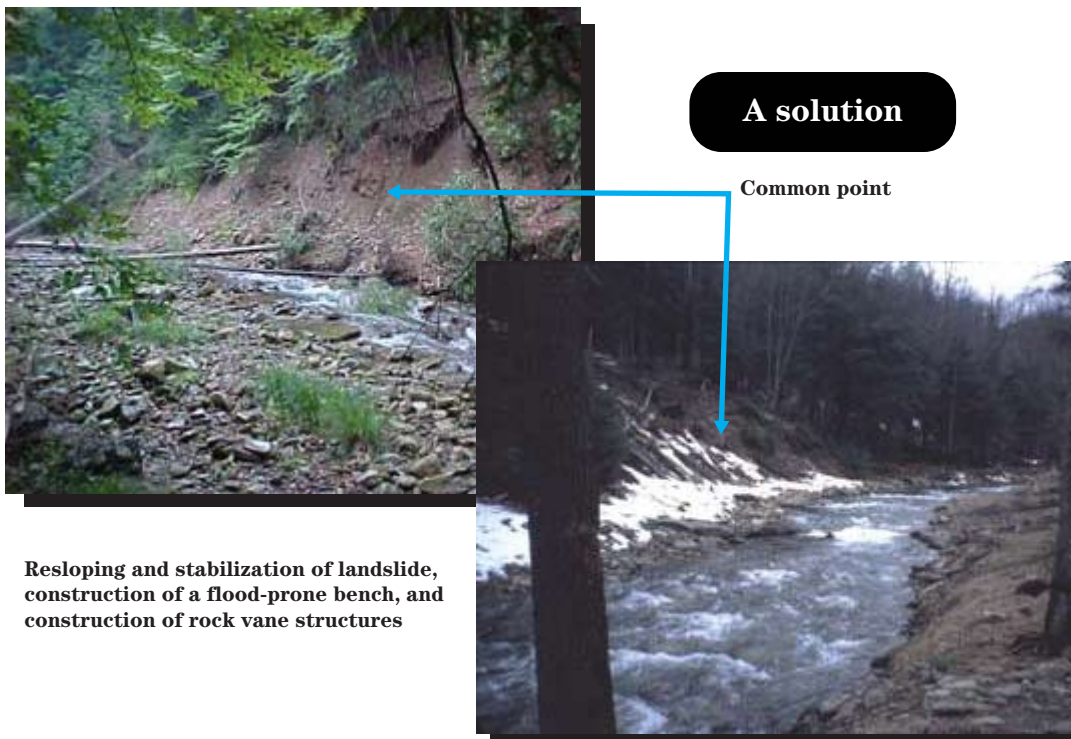
Figure CS6-20 Treatment technique used for a landslide area
