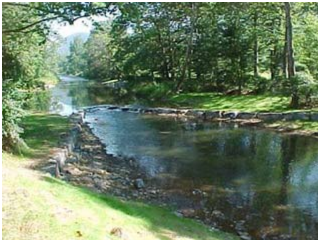
Figure CS6–17 Cross vane illustrating the proper upstream fill along the vanes, leaving a flat horizontal ramp along the vane
