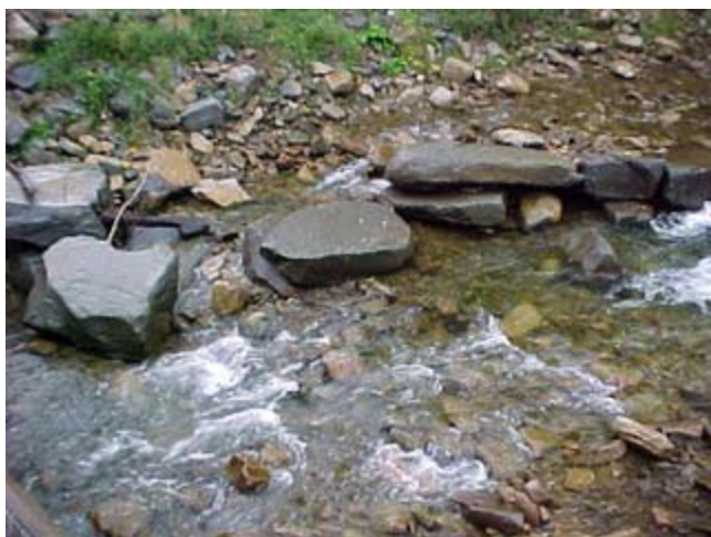
Figure CS6-12 Example of vane rocks with small footer rocks and inadequate long-term performance
