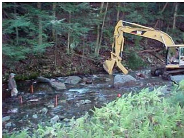
built the structure using the eyeball technique. That is, the structure was built by an operator substituting a trained operator eye for the use of a construction transit or laser level. Consequently, the slope along some of the problem structures measured greater than 7 percent (or even 10%), as constructed.
