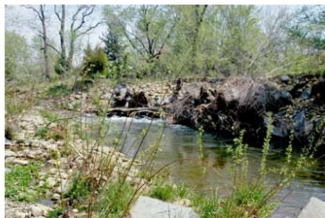
Figure CS5-16 Upper rootwads, April 2004, after Hurricane Isabel
