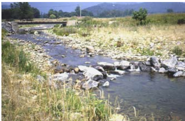
Figure CS5-4 Weir #7, July 1998
