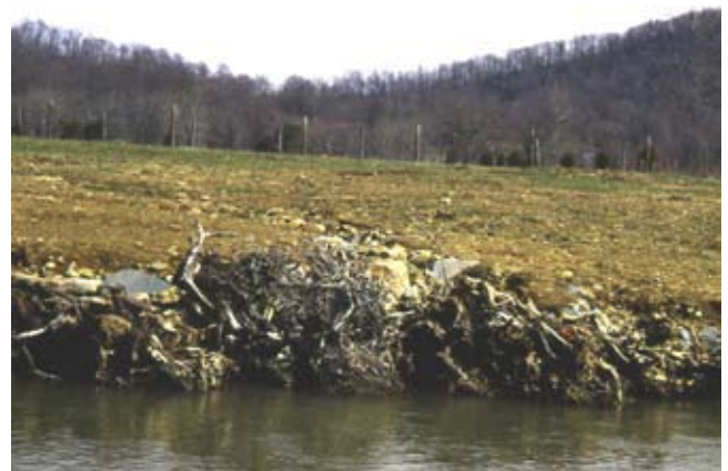
Figure CS5-3 Lower rootwads, March 1998, immediately after construction
