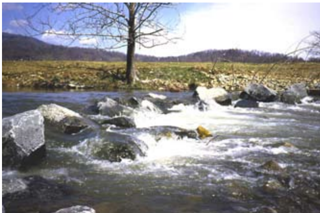
Figure CS5-2 Weir #5, March 1998, immediately after construction
