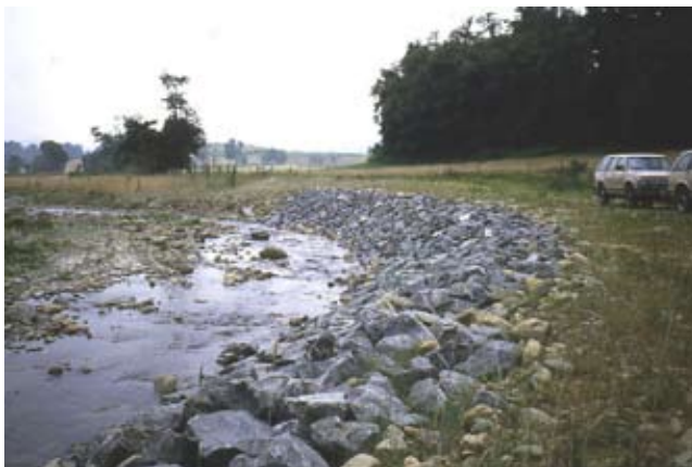
Figure CS5-6 Upper riprap, July 1998, 3 months after construction
