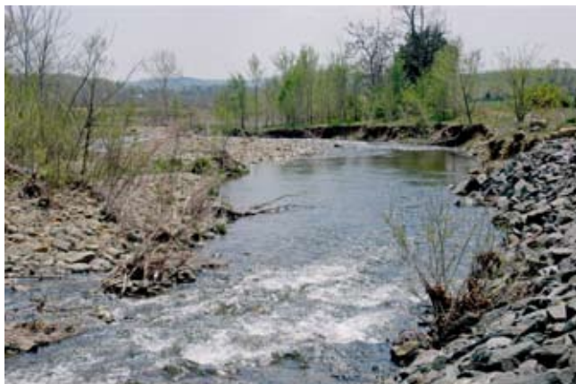
Figure CS5-15 Raw bank downstream of riprap
