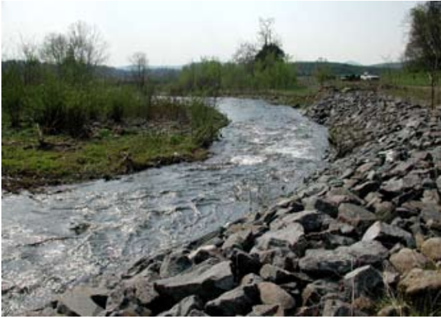
Figure CS5-8 Upper riprap, April 2003
