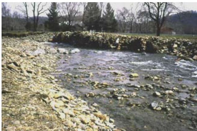
Figure CS5-5 Upper rootwads after construction, July 1998
