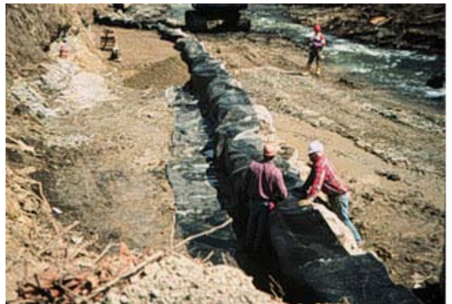
Figure CS4-9 Primary geotextile anchorage length
