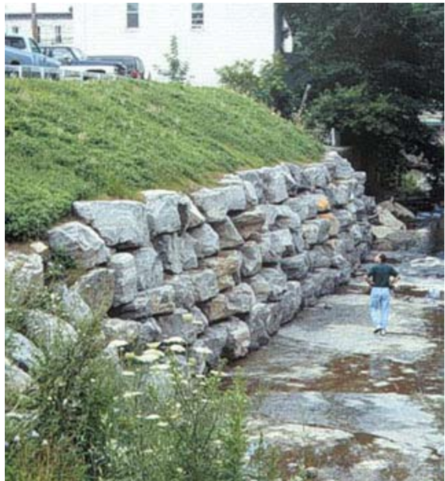
Figure CS4-13 Completed wall
