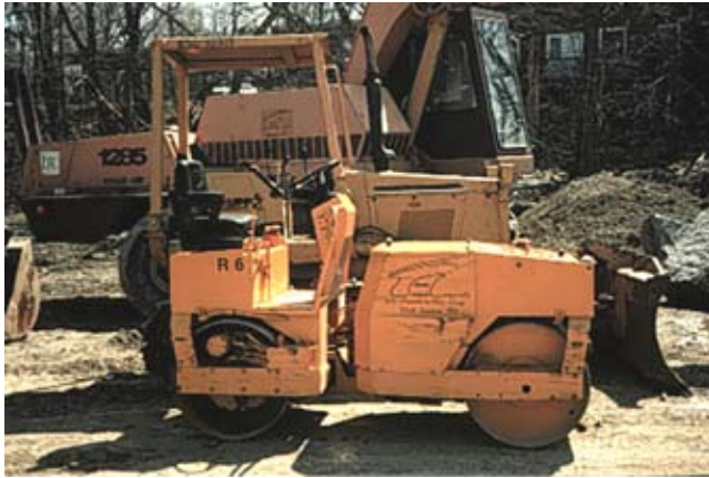
Figure CS4-6 Compaction equipment
