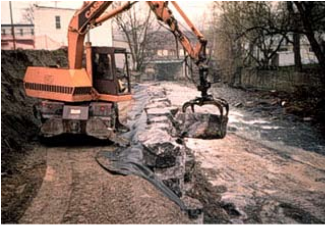
Figure CS4-10 Stacked riprap face placement
