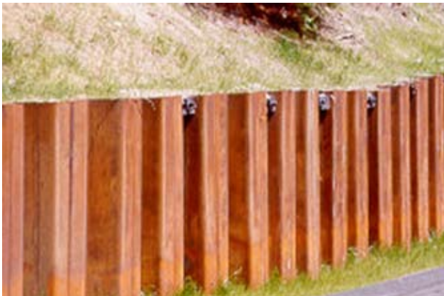
Figure CS4-1 Sheet pile wall
