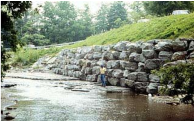
Figure CS4-12 Completed wall
