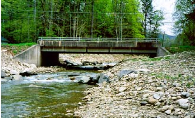
Figure CS4-4 Concrete wall alternative
