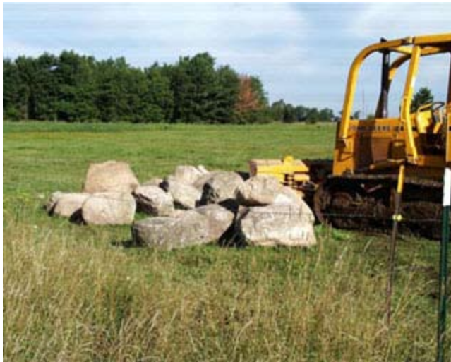
Figure CS3-10 Boulders used for random placement in the stream
