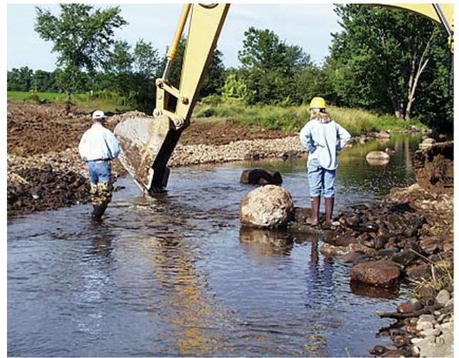
Figure CS3-11 Random boulder placement with DNR fish manager and NRCS engineer
