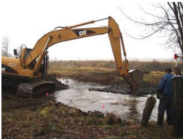
Figure CS3-5 Removal of rock dam crossing, Nov. 2001
