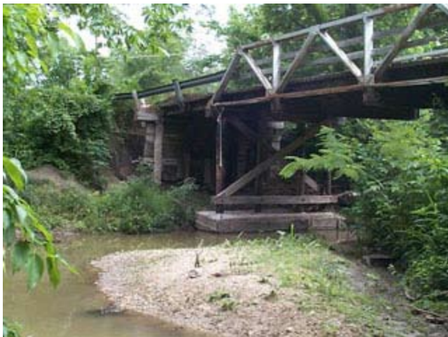
Figure CS2-1 Original timber-plank bridge structure
