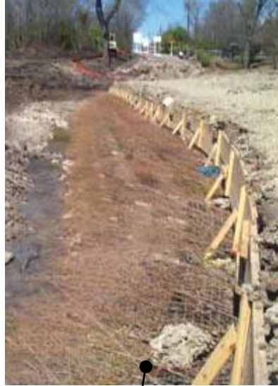
Figure CS2-4 Vegetated geogrids and dormant post plantings are the two primary streambank soil bioengineering measures.
