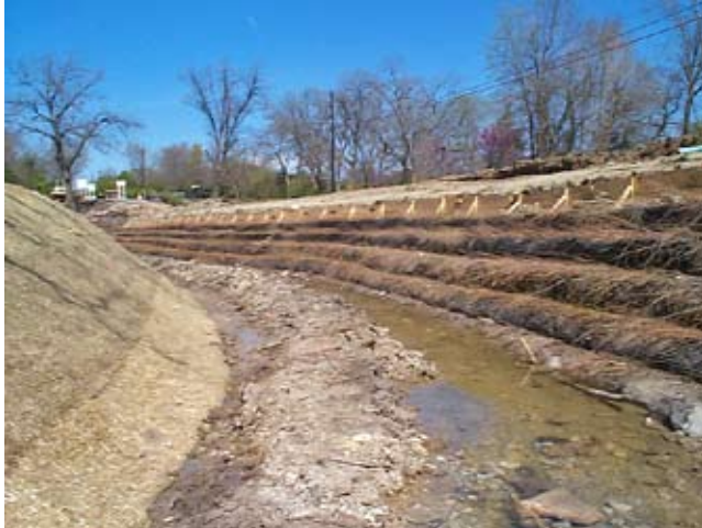
Figure CS2-7 (a) Mar. 2001—Goode Road embankment was stabilized with vegetated geogrids. The opposite bank on the left was protected with soil erosion blankets; (b) Apr. 2003—biomass increases with time; (c) May 2002—black willow covered the entire bank 1 year after construction.
