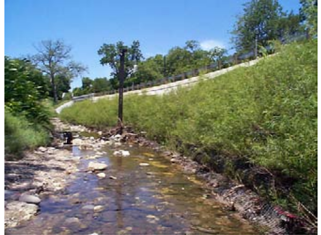
Figure CS2-7 (a) Mar. 2001—Goode Road embankment was stabilized with vegetated geogrids. The opposite bank on the left was protected with soil erosion blankets; (b) Apr. 2003—biomass increases with time; (c) May 2002—black willow covered the entire bank 1 year after construction.
