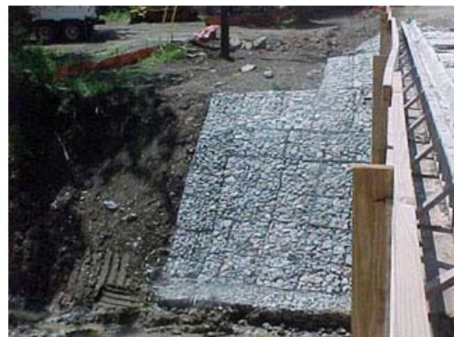
Figure CS2-3 Gabion mattress was used for the bridge abutment area.
