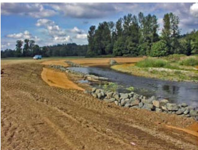
Figure CS17-9 Looking downstream at completed project showing barbs and erosion control mat during summer flow ( Photo courtesy of Scott Wright )
