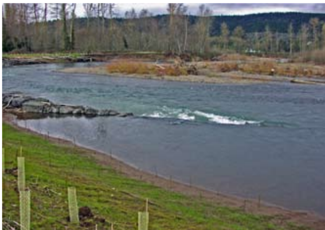
Figure CS17–13 Example of energy dissipation from a hydraulic jump formed over one of the project barbs during winter baseflow (Photo courtesy of Scott Wright)
