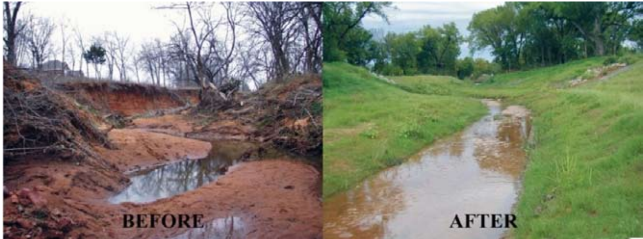
Figure CS16-11 Eroding channel prior to construction and after project implementation
