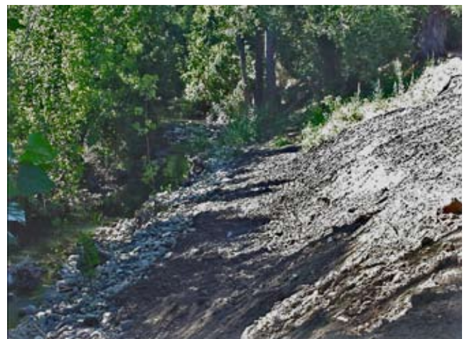
Figure CS15-6 Cobble placement following the live siltation installation
