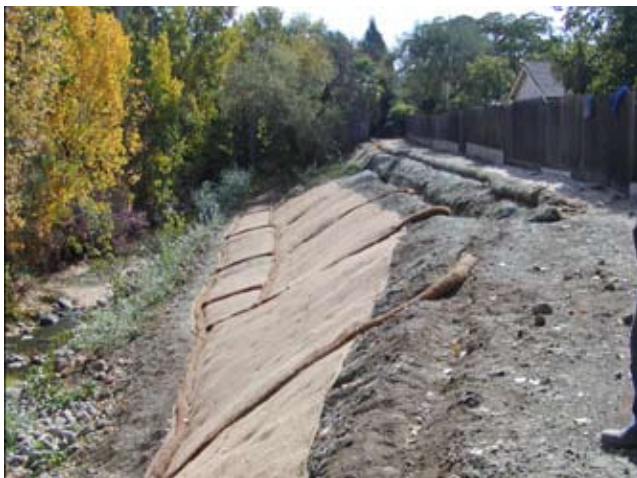
Figure CS15-8 Slope preparation and blanket installation
