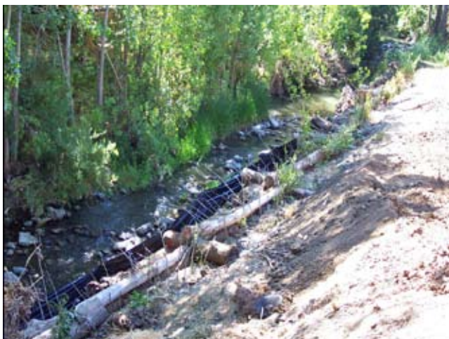
Figure CS15-5 Live siltation installation
