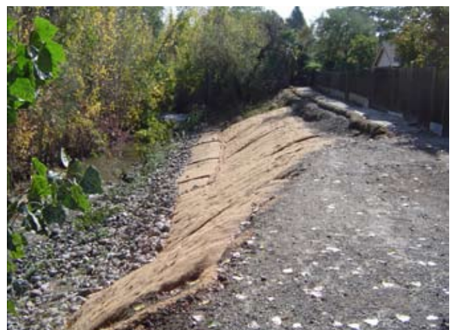
Figure CS15-9 Finished project
