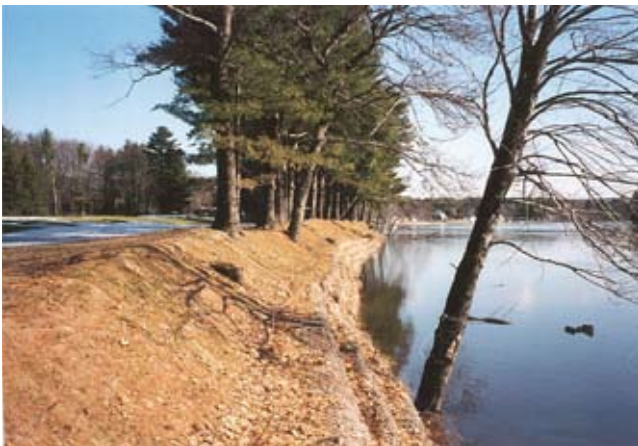
Figure CS14-9 Project in spring after initial installation
