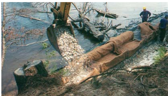
Figure CS14-8 Installed gabion baskets lined with coconut fiber mat and filled with stone and topsoil
