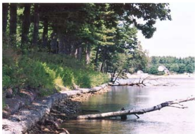
Figure CS14-10 Completed project in midsummer after installation
