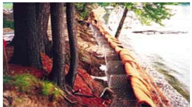
Figure CS14-8 Installed gabion baskets lined with coconut fiber mat and filled with stone and topsoil
