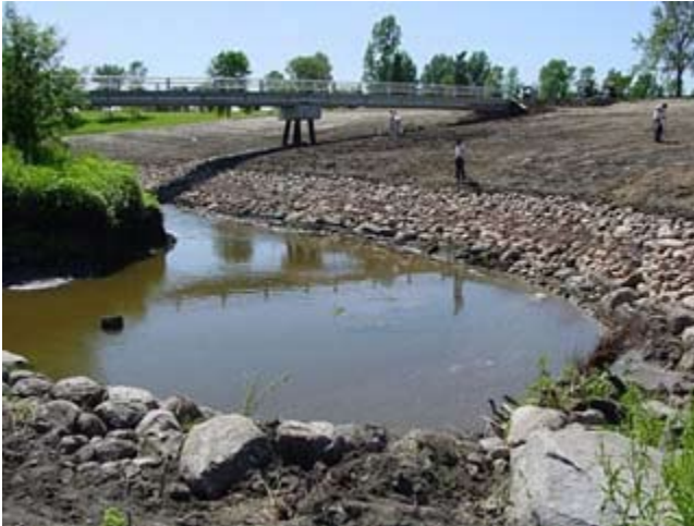
(a) Looking upstream toward the cart bridge
