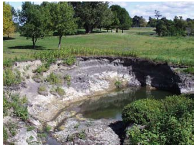
Figure CS11-8 Looking downstream on Cole Creek at the scour erosion caused by the narrowed channel
