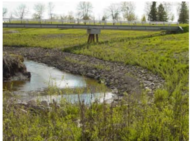
(b) Looking upstream toward the new golf cart bridge
