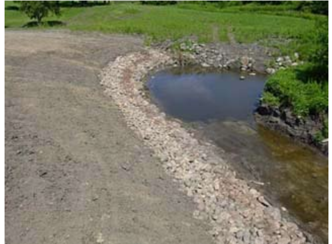
(b) Looking downstream from the cart bridge
