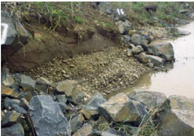
Figure CS10-6 Fitzgerald site, photos taken from similar view points. Initial erosion at toe adjacent to RB; structures filled with sediment as vegetation developed
