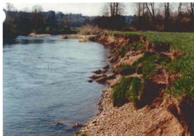
Figure CS10–1 Typical conditions that existed at the project sites prior to design treatments
