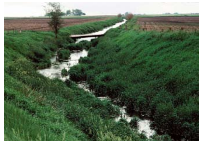
Figure 10-2 Drainage ditch constructed in north-central IA
