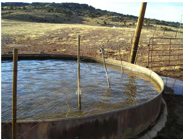
**Figure 2** Braces across trough made of wire or steel bars
