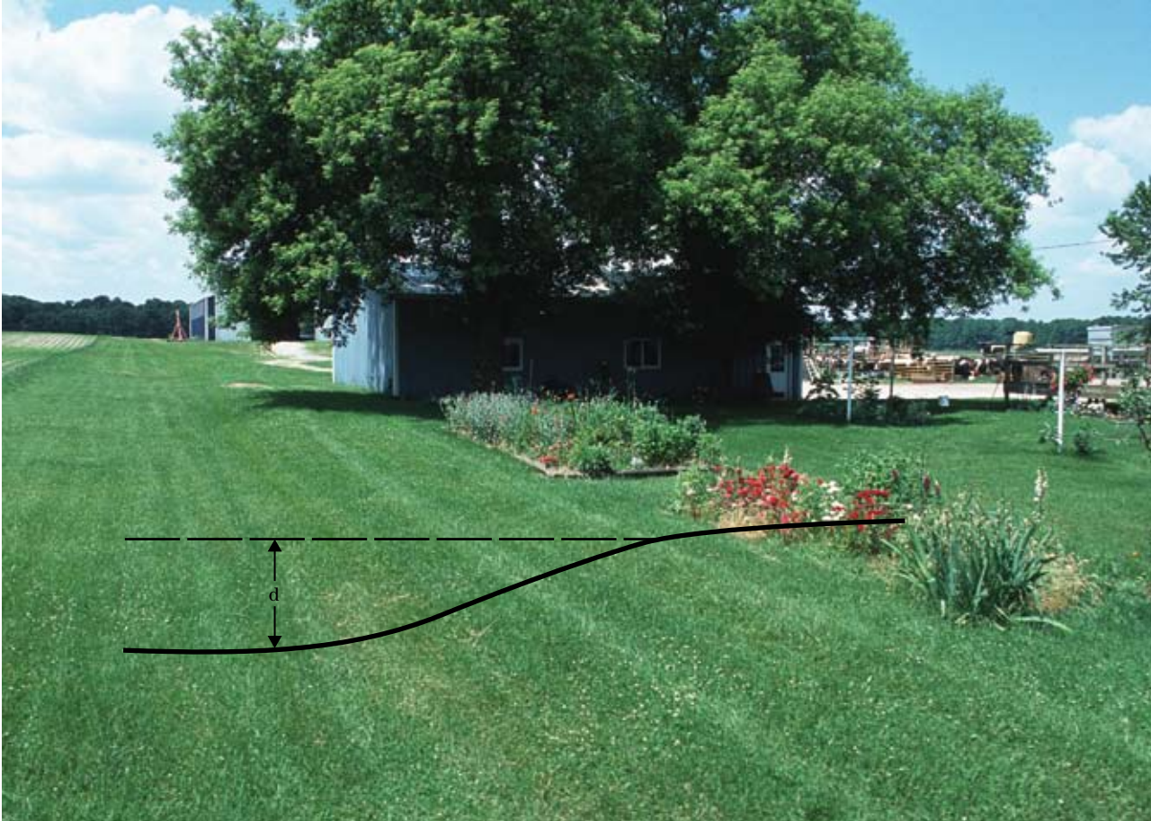
Figure 9-1 Typical diversion
