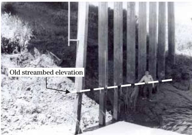
**Figure TS3B-4** An NRCS bank stabilization site that did not include streambed stabilization, (Page County, IA)
