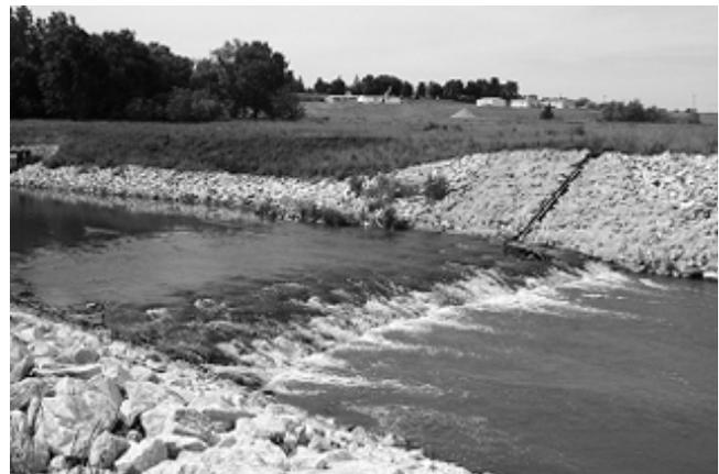
Streambed stabilization structures have many benefits. They decrease the slope of the streambed, reducing water velocities. They prevent further downcutting, protecting farmland, bridge pilings, and utility lines from future erosion. They create an upstream backwater condition which allows sediment to settle out, reducing sediment loads and improving water quality. The backed-up water often helps to protect bridge pilings by submerging them.
