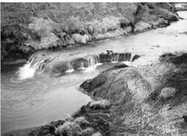
**Figure TS3B-5** HCA steel sheet pile weir with riprap and cement grout that protects a large sewer main for the City of Denison, IA
