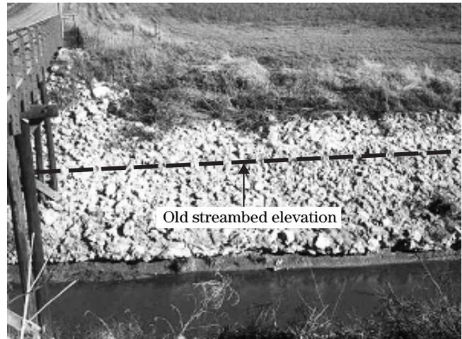
**Figure TS3B-3** Nickpoint eroding headward
