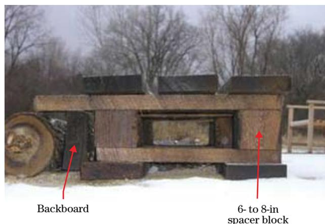
**Figure TS140-5** LUNKERS construction concept plan
