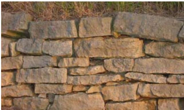
A sloping bench can be provided behind the wall to serve as a transition slope on which vegetation can be planted. Well tamped backfill should be placed behind the wall and in the spaces between the rocks as they are placed. Live branch cuttings can be placed in the interstices of the rock wall as it is constructed. The butt ends of the branches should extend into the backfill behind the wall. A cross section of a vegetated rock wall is shown in figure TS14M-2.
