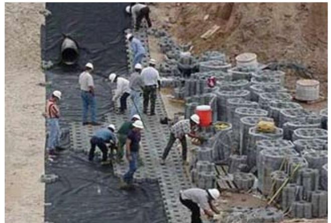
**Figure TS14L-20** ACB termination trench
