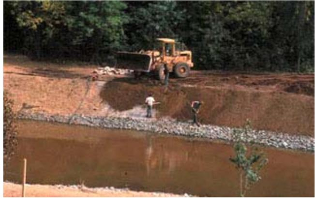
**Figure TS14L-22** ACB revetment system 1 year after completion (*Photo courtesy of Joe Polulech*)
