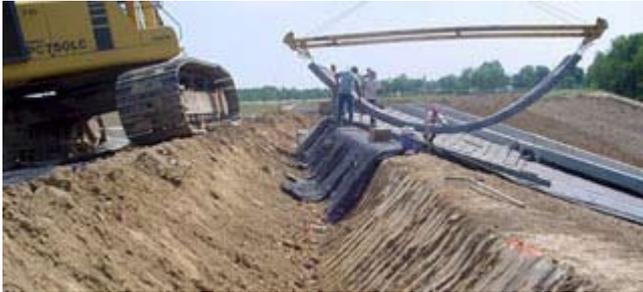
**Figure TS14L-21** Filling ACBs with top soil (*Photo courtesy of Joe Polulech*)
