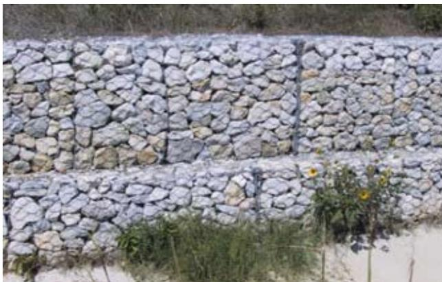
**Figure TS14K-12** Vegetated gabions under construction
