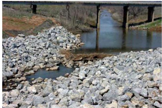
**Figure TS14C-3** Riprap used to prevent erosion from flow from a side inlet to a channel
