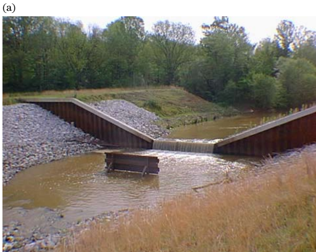
Figure TS14B-18 (a) Low- and (b) high-drop grade control structures
