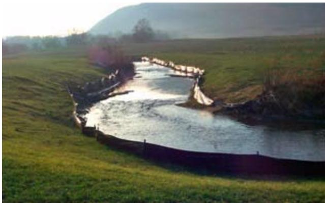
**Figure CS7-7** Completed section of streambank stabilization to include J-hook vane and intentional point bar, Spafford Creek, NY
