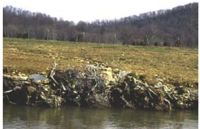
some time in the past, large slabs of concrete had been placed along the river. These were used as the footers for the first four or five rootwads. Large logs were used as footers for the remaining rootwads. Approximately 60 tons of Class III riprap was placed over the boles of the rootwads at the lower end of the set. These were covered by soil.
