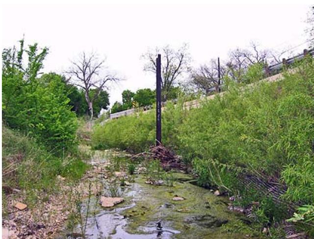
**Figure CS2-8** (a) May 2001—dormant black willow posts installed on the first creek bend. Rocks were used to protect the toe area; (b) Nov. 2002—black willow covered the bend 1 year after construction.
