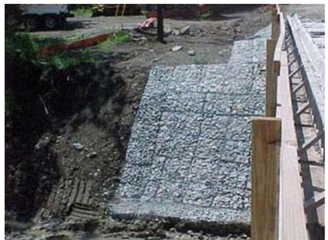
**Figure CS2-4** Vegetated geogrids and dormant post plantings are the two primary streambank soil bioengineering measures.
