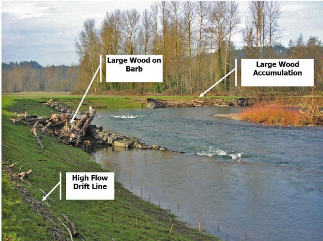
Detailed topographic information was collected pre- and postconstruction to identify actual geomorphic effects of the stream barbs and overall performance. Figure CS17-12 identifies the actual scour that occurred around each barb and the streambed.
