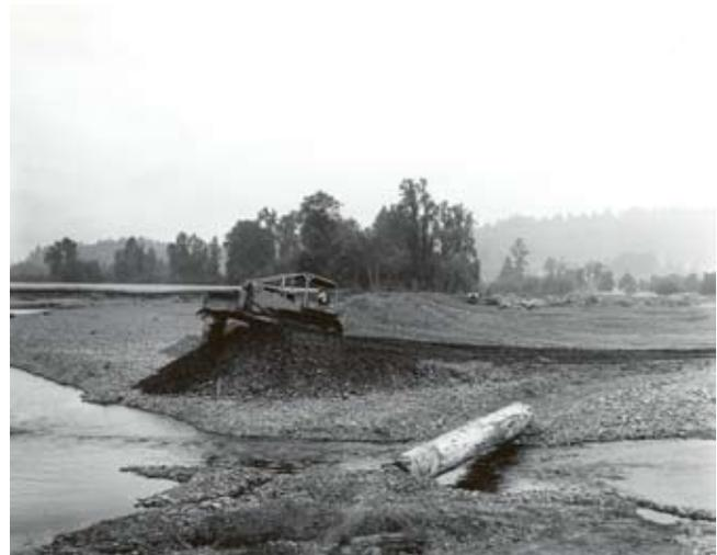
**Figure CS17-3** Aerial view of project area in 1966 showing dikes used to cut off meanders
