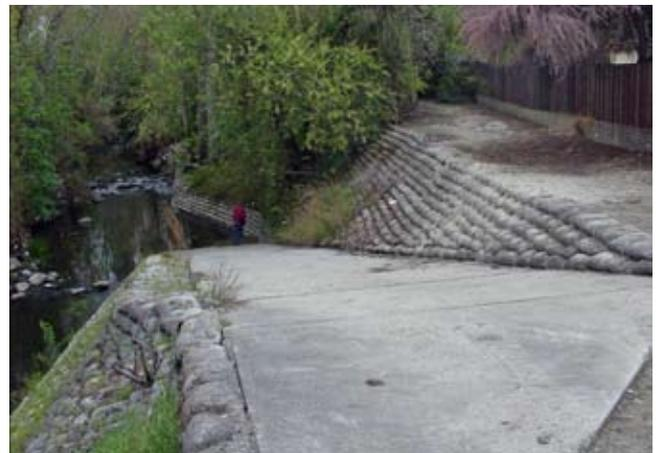
the bank including vegetated log cribwall structures, geotextile erosion control blankets, and native vegetation. The primary goal was to protect the integrity of the downstream bridge while providing shade, wildlife habitat, and local bank stability.
