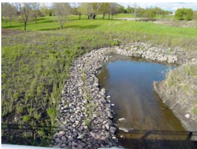
(a) Looking downstream into the meander
