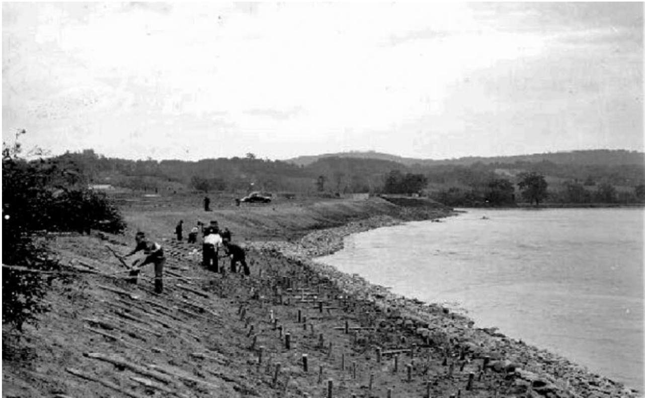
Figure E-2a Streambank soil bioengineering techniques
