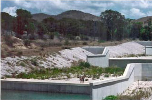
**Figure 7-2** Grass-lined threshold channel
