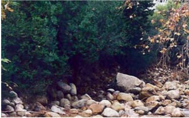
**Figure 7-8** Subsurface layer exposed after removal of three cobbles from the armour layer
