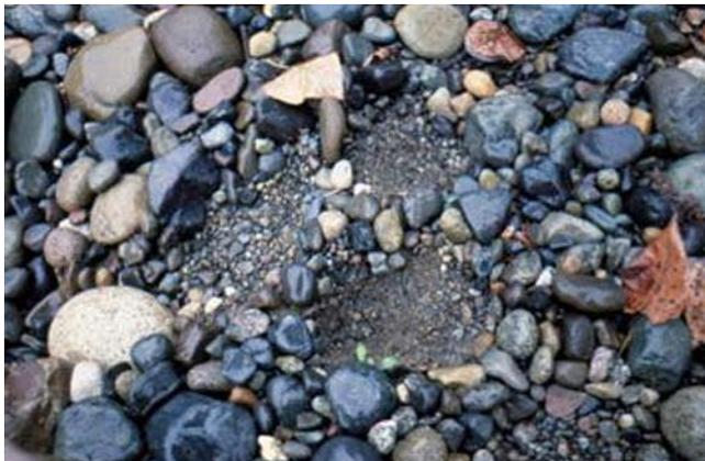
**Figure 7-9** Degradation through armor layer
