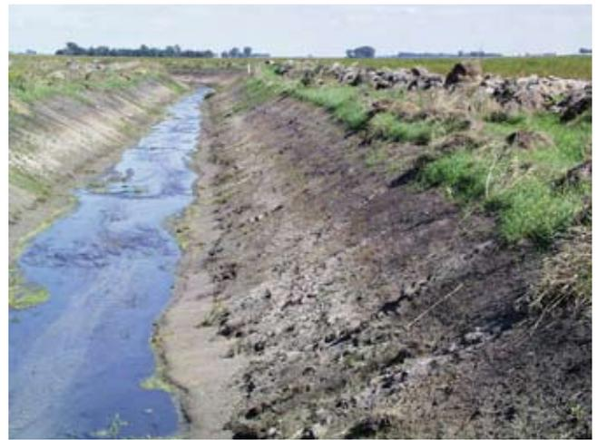
**Figure 10-5** Two-stage ditch geometry with minimum sized benches
